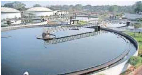
Once all the new plants become operational, the treatment capacity would almost double. Express
